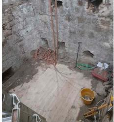
Above: It was cold working in the tower of St Cuthbert's Church in November (photo John Halsey) Left: Old belfry floor removed and making ready for the new joists and bell frames (photo Nick Ward) Below left: Removing the wheels Below right: And the treble makes three (photos Nick Ward)
