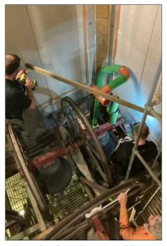
Suspending the newly constructed ducting from a wooden baton placed diagonally above the treble pit
